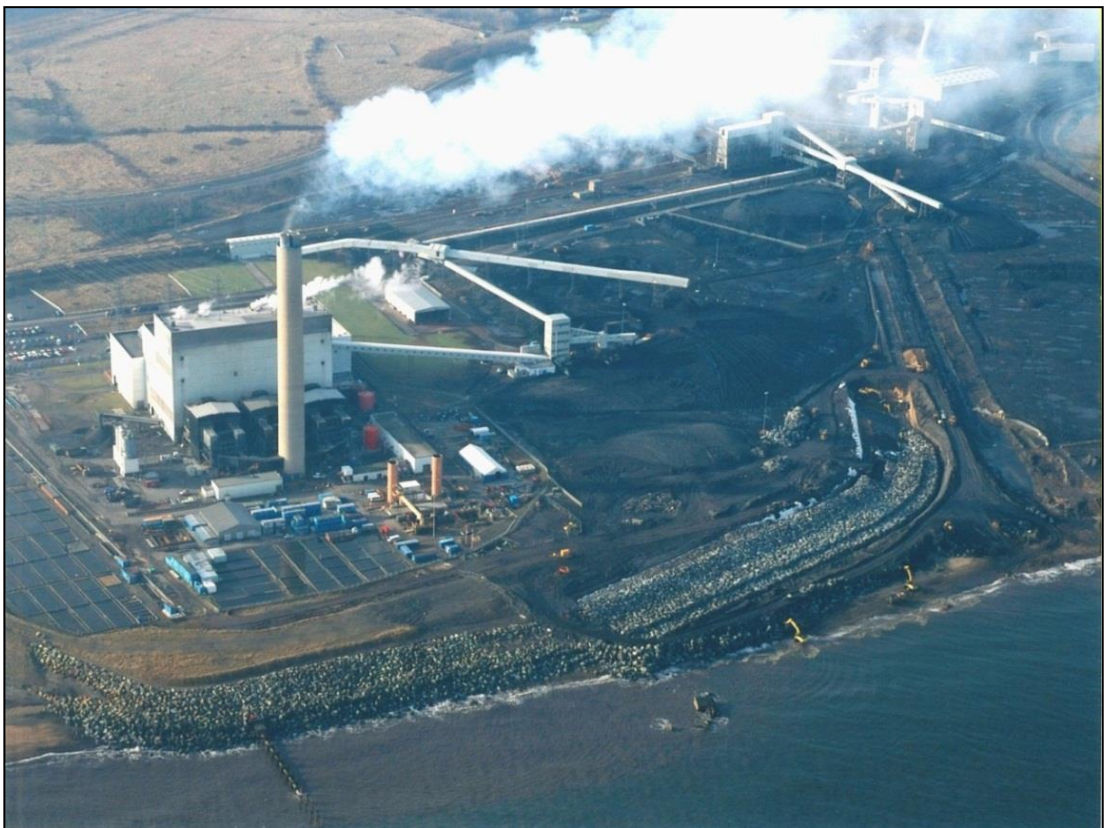
Figure 3 – Coastal Defences at Lynemouth Power Station
